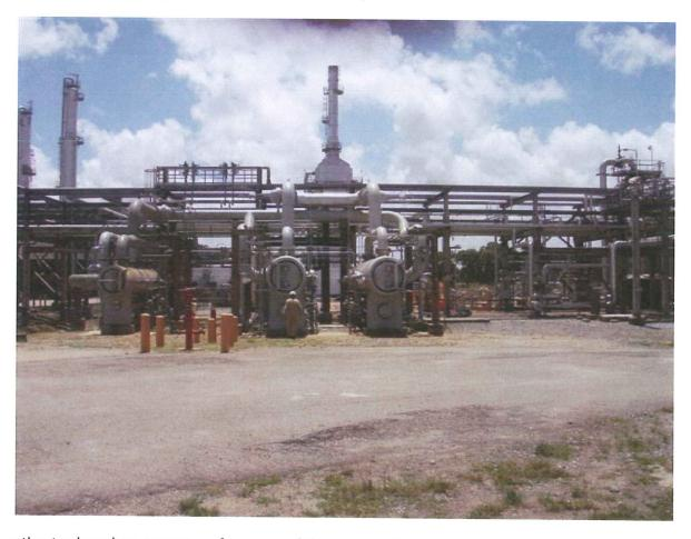
PPGPL estimates based on current performance of the regeneration cycle, a 4-5 year molecular sieve bed life. Black & Veatch purchased two 68" Sepra-Chem Dual Closure Coalescers for PPGPL's Phase 3 under construction in 2007 designed at 660 MMSCFD. PPGPL plans to purchase additional Sepra-Chem Coalescing equipment to replace existing Phase 1 coalescers. Please contact Sepra-Chem Corporation at 903-566-1015.
